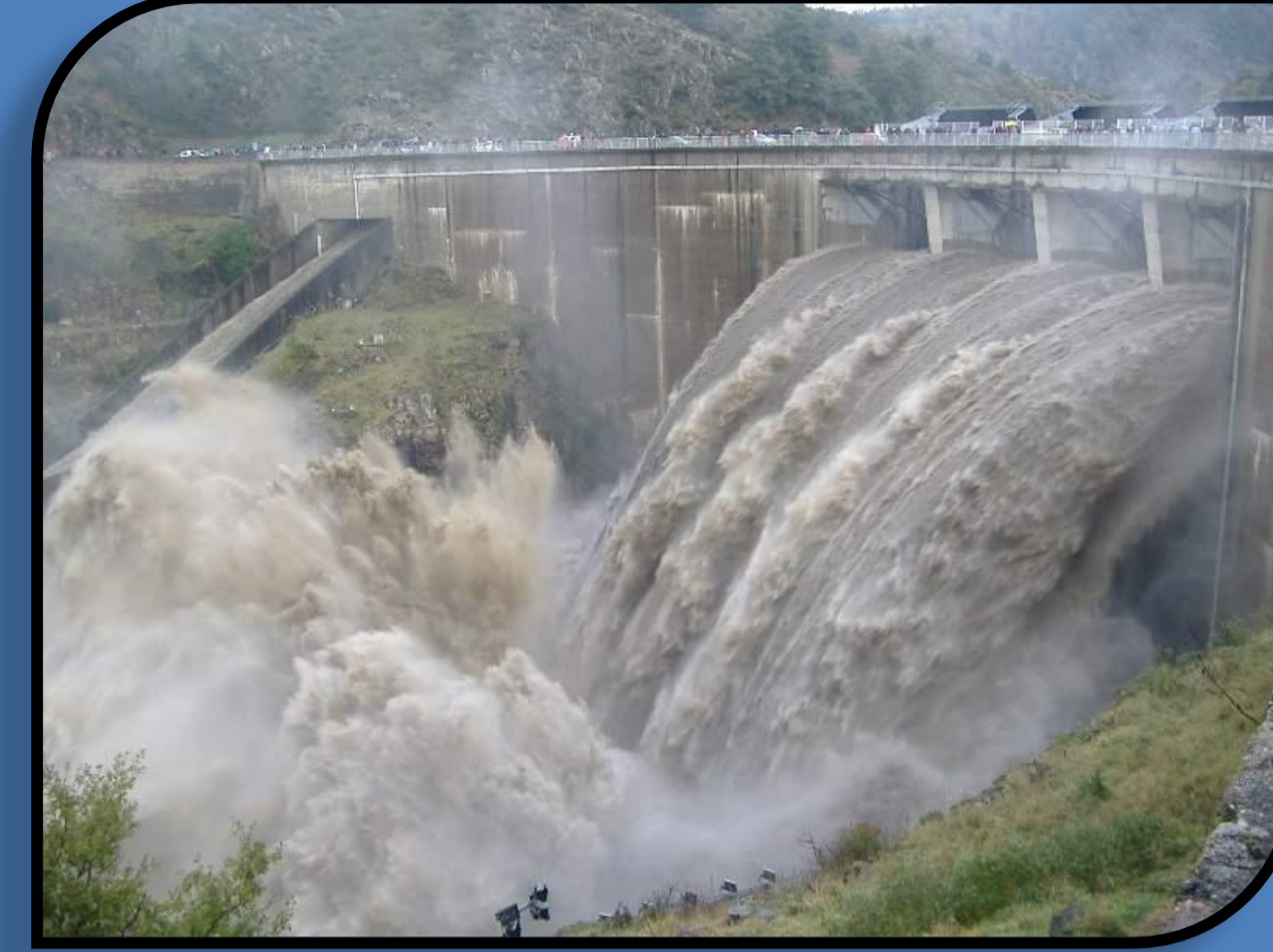
Loire at Grangent, november 2008.
